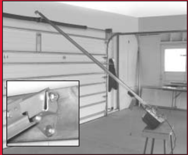
FIG. 2-7 Position assembly.
