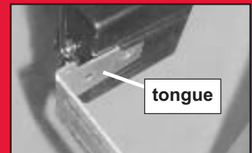
FIG. 3-3 Attaching "STB's" to brackets.
