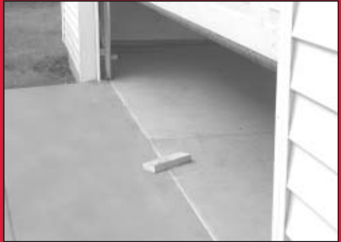
FIG. 7-5 2 x 4 under center of door opening.
