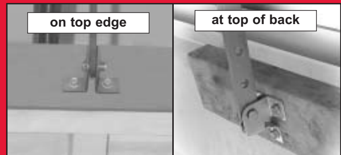
FIG. 2-7B Mounting door Bracket (one-piece).
