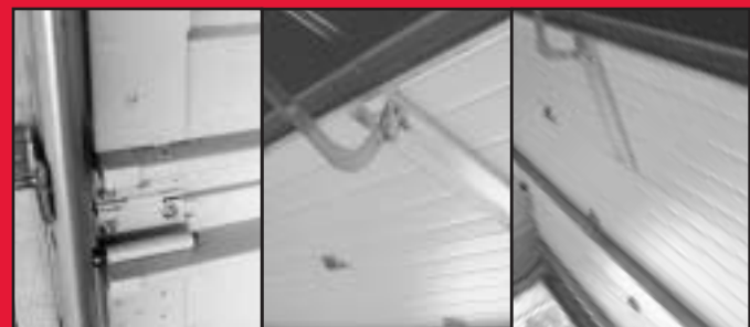
FIG. 2-6 Examples of door bracing.
