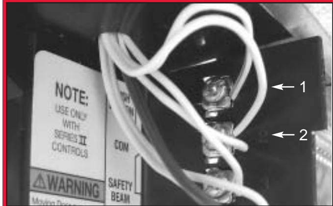
FIG. 5-1 Terminal attachments at power head.
