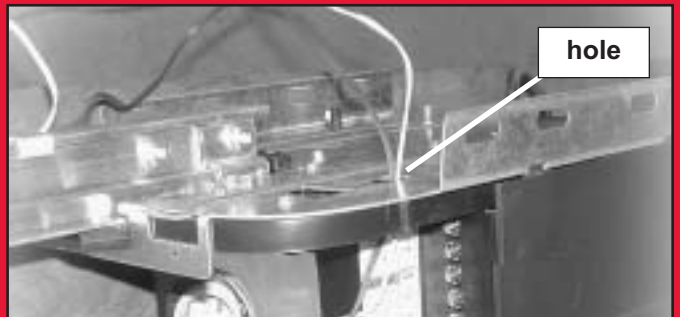
FIG. 1-8 Run wire to power head.
